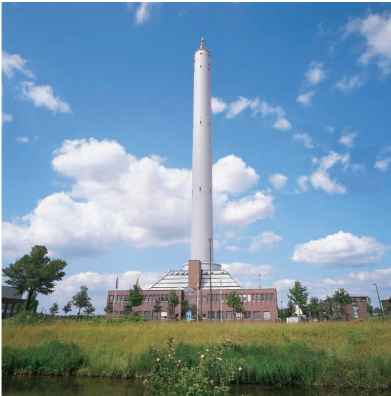
Figure 5: Drop tower of the Center of Applied Space Technology and Microgravity (ZARM) with a height of 146 m (courtesy of ZARM).
